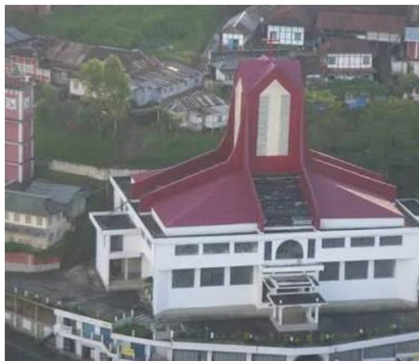
Pic 10: MTBA constructed in 1980s
